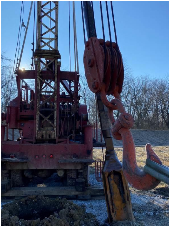
Photograph submitted by Hugh Downer, CPG 11815. Photograph taken in February 9 2024. Installing Large Diameter Public Water Supply Well Using Cable-Tool Drilling, Columbus, Ohio.
